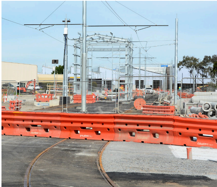
Entrance to the new Maidstone Depot, 6 December 2024.
